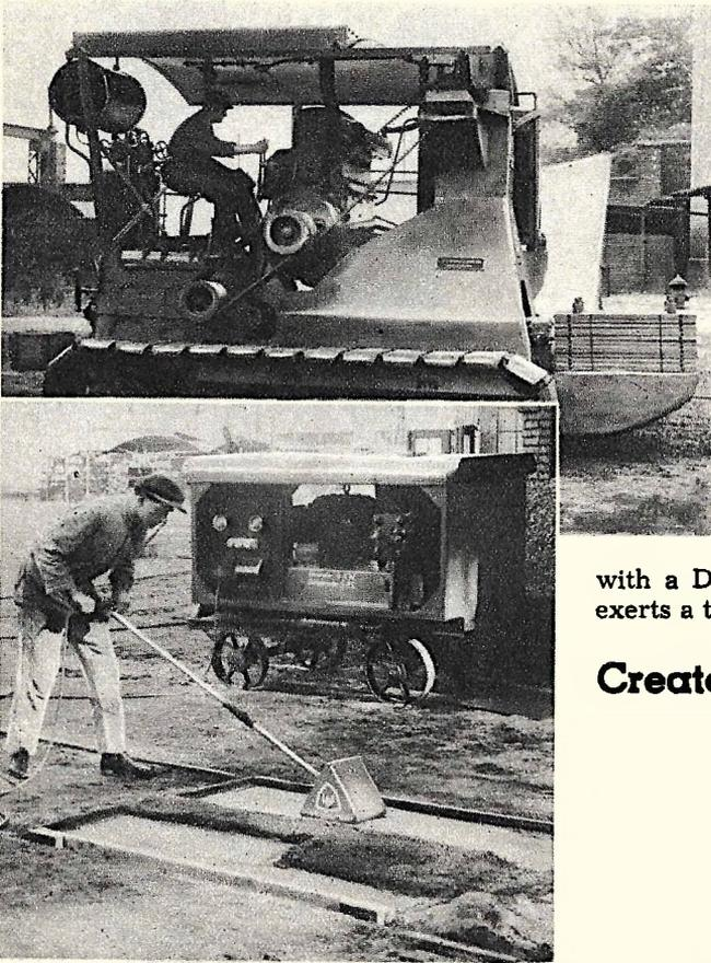
Top—Equipped with a 100-horsepower Diesel engine, this machine tamps down new asphalt and concrete roads with a tamping pressure of 60,000 pounds. Bottom—This hand operated tamper exerts 600 pounds pressure.
