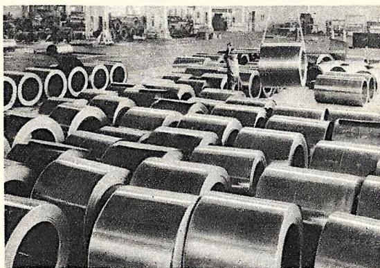
The finished product ready for cold-forming into auto bodies and hundred-and-one other products. It is shipped in flat sheets, as at left, and in coils weighing tons each.
