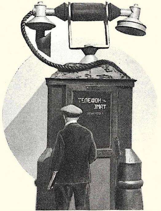
Telephone pay stations aren't difficult to locate in Russia. Giant hand sets like this one have been erected on the roofs of phone booths to popularize service. Phones are of sheet metal.
