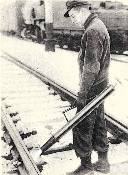
Developed in cooperation with the U. S. Forest Service this gasoline blow torch has an overall length of 41 inches. It is used to destroy weeds along tracks and to thaw frozen switches.
